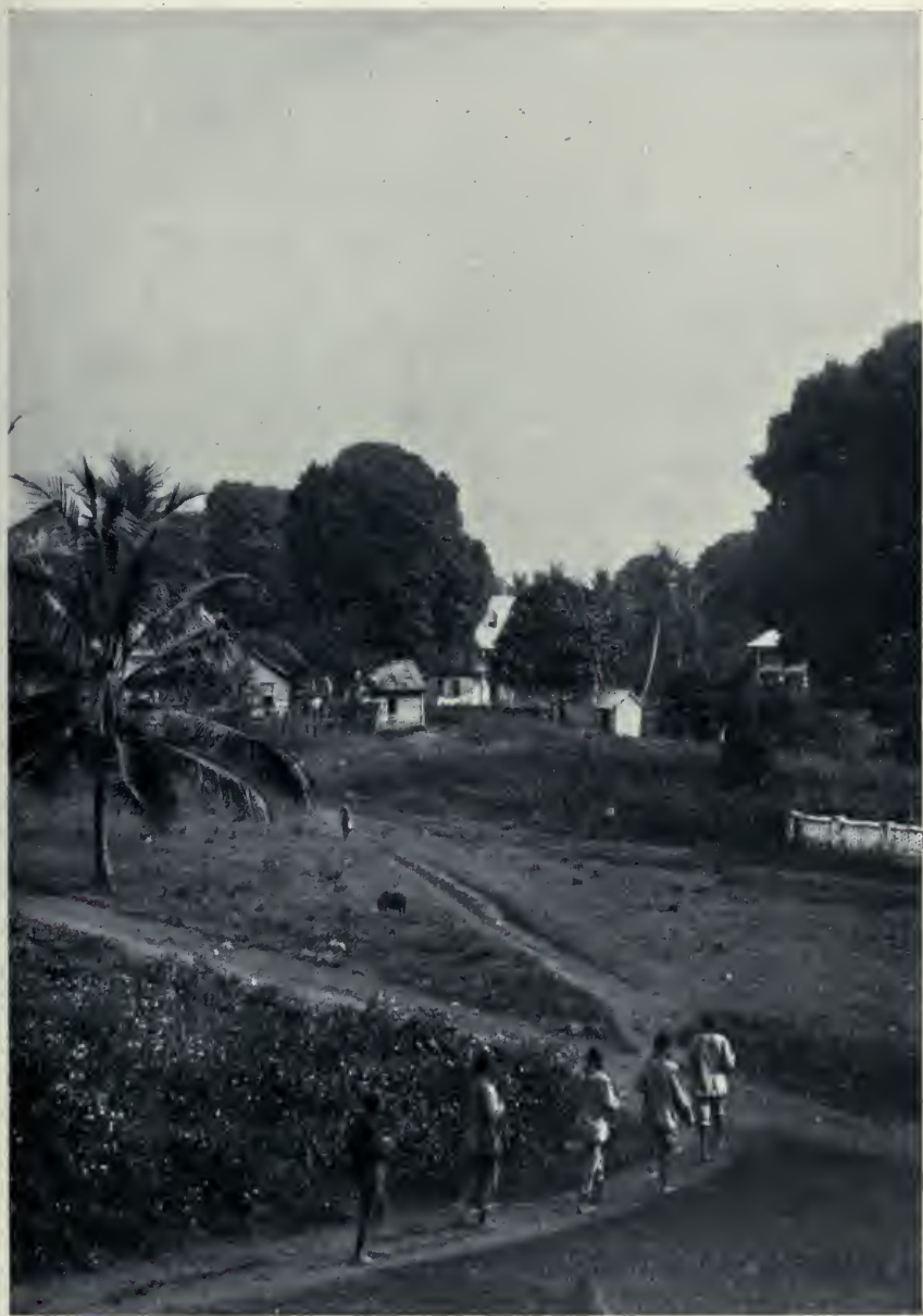
182. ON THE OUTSKIRTS OF MONROVIA
