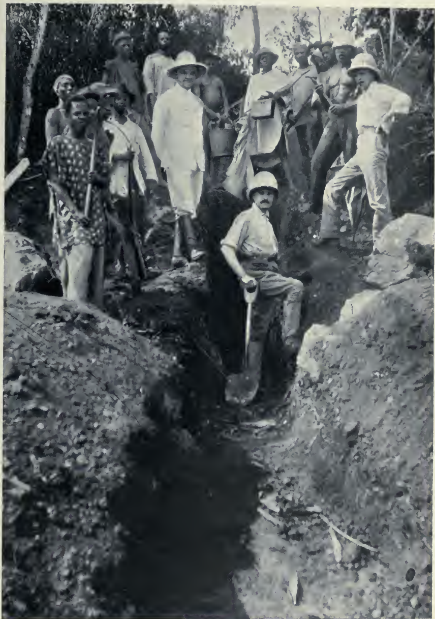
208. SINKING A SHAFT IN A QUARTZ REEF NEAR THE ST. PAUL'S RIVER
