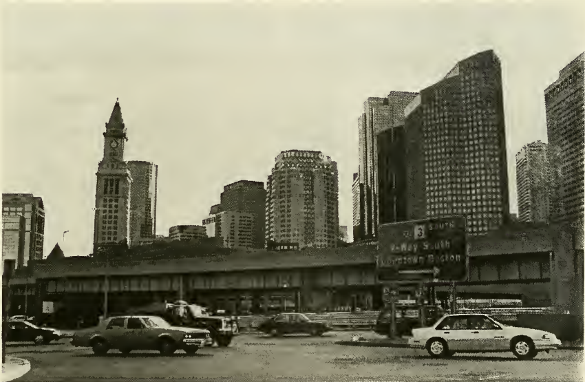
View of Central Artery from North End Custom House Tower and Government Center in background
