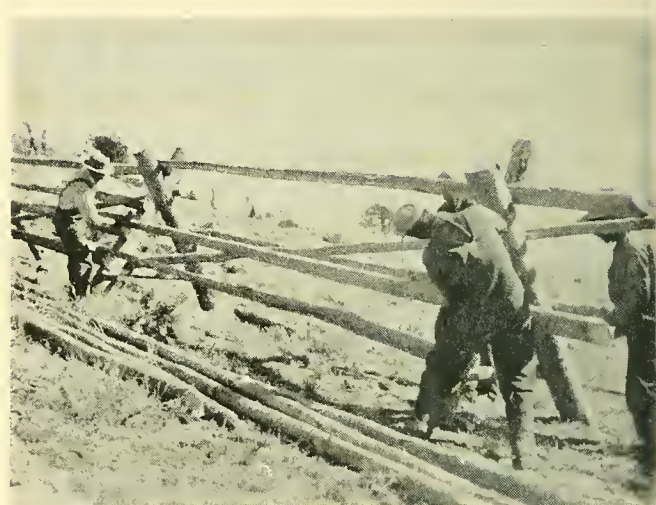
Drift Fence To Conserve Snow For Stock Water, Shoshone. Over 100 miles of Range Fence Had Been Built By IEC Workers On Reservations By October 1, 1933
