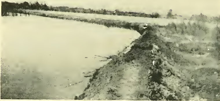
A Dyke Made By Indian Crews Holding The Water In Fields That Were Once Waving Stands Of Johnson Grass
