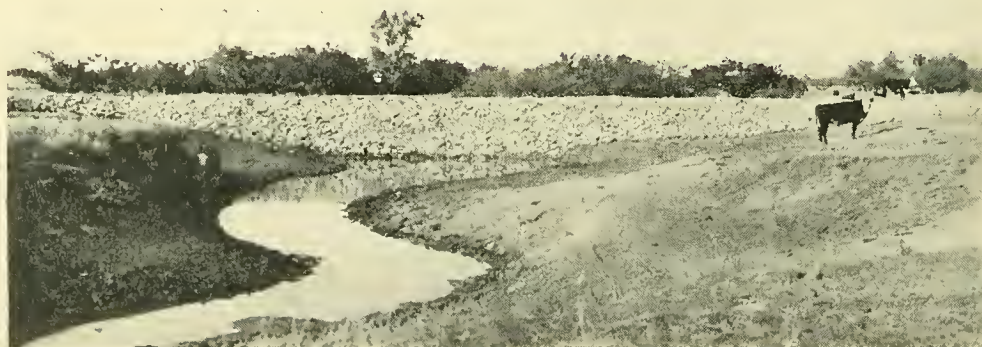
A Dam To Save Soil, Kiowa Agency. A Structure To Provide Stock Water And Check Erosion
