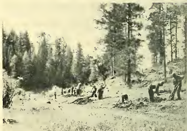
Fire Trail Work. Pima Indians At Ft Apache
