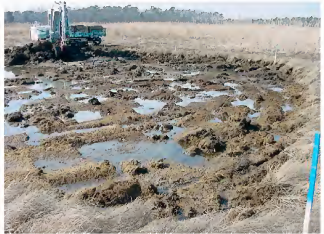
Figure 4: High marsh, vegetated with Spartina patens , is chosen to be sacrificed in the OMWM excavation. Note that the invasive Phragmites australis is left in place. From Figure 16, page 130 of the Memoirs (image credit: Suffolk County Department of Public Works).
