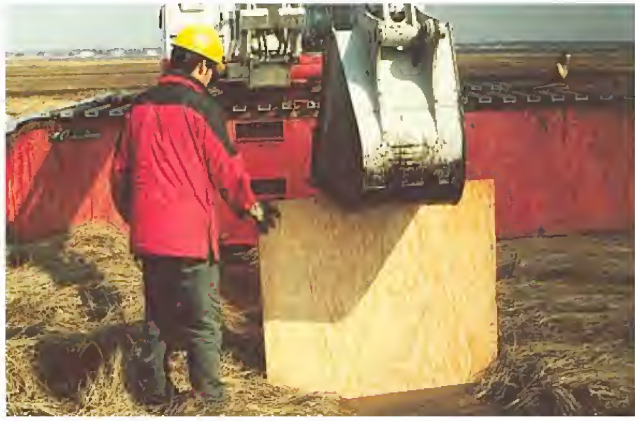
Figure 2: A piece of plywood being knocked into a ditch with the bucket of a backhoe. The plywood acts as a plug. The blocked ditch ceases to serve as an artificial channel for marsh drainage, and as a result, large ponds can form on the marsh (behind the blocked portion of the ditches). Figure 39, page 140 of the Memoirs (image credit: National Park Service).
