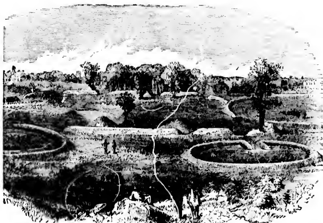
View of Earth-works at Hopeton.
